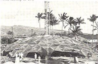
Part way through, the dome begins to assume its characteristic shape. Panel installation was completed in just 20 hours.
