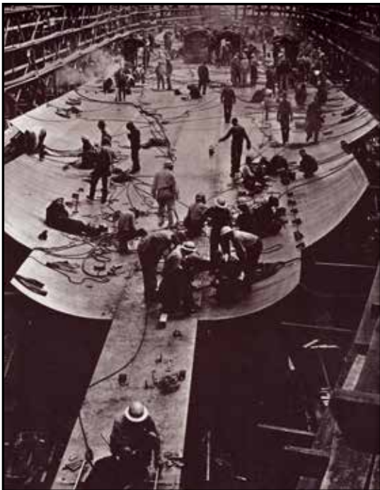
Welders swarm over a newly-laid keel to join the steel plates at the Kaiser Shipyards in Richmond, CA.
