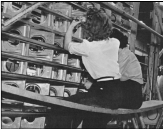
At the Fleetwings plant in Bristol PA, female war-workers make final adjustments on a B-17 bomber fin.
